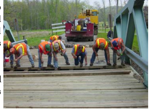
Structure 1265-2260 on TR 1265
