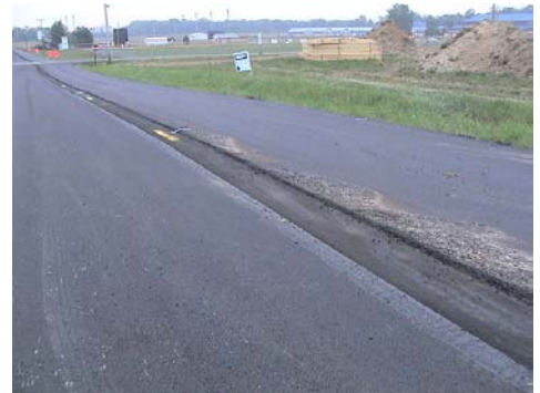
Paving project on CR 620
