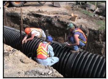
Culvert Repair by County Work Force
