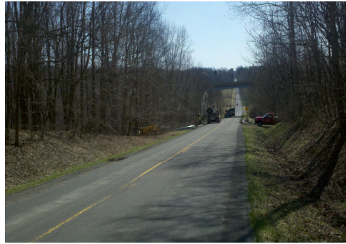
County Road 1035 Guardrail
