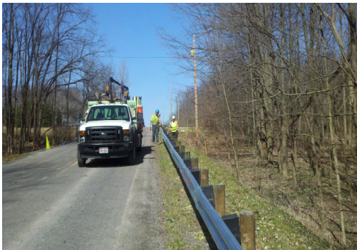
County Road 1035 Guardrail
