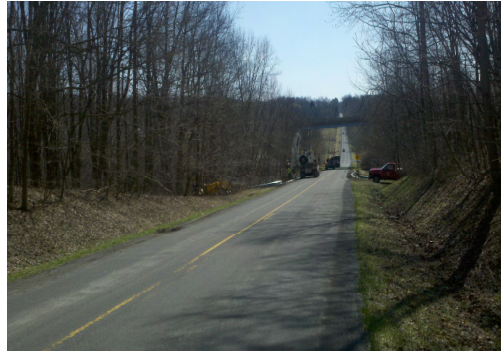
County Road 1035 Guardrail
