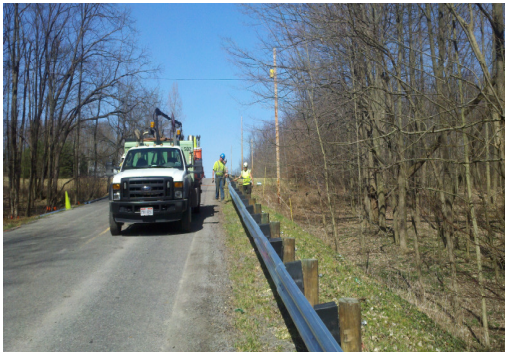
County Road 1035 Guardrail
