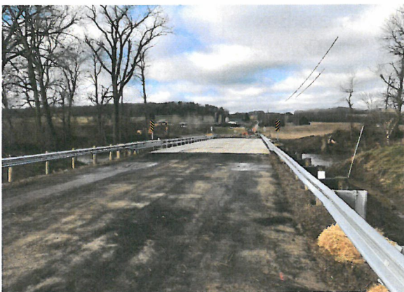
Bridge 2575-170-Lake Township
