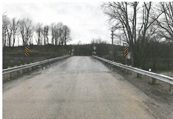
Bridge 1075-2525-Green Township
